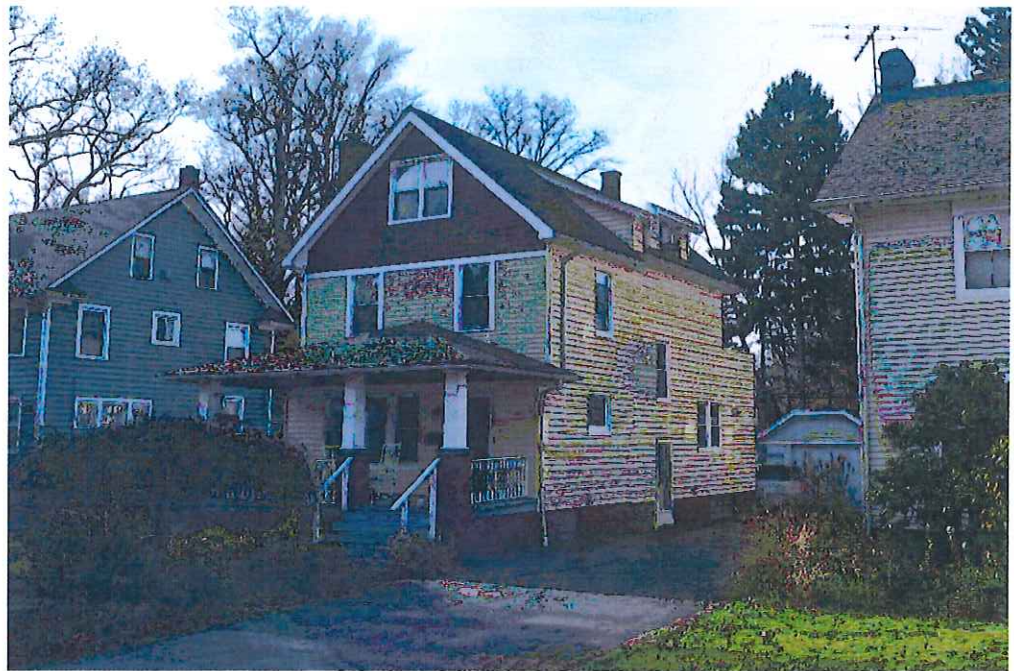
View Looking Southwest
