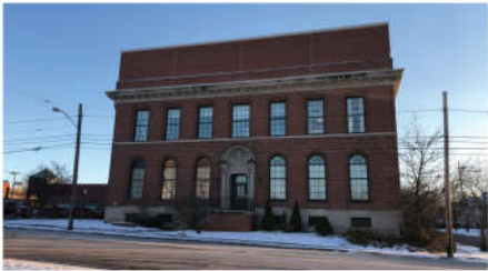
B At&T Building
