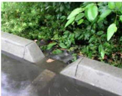
FIGURE 1166.06(b)(6): EXAMPLE OF CURB INLET
