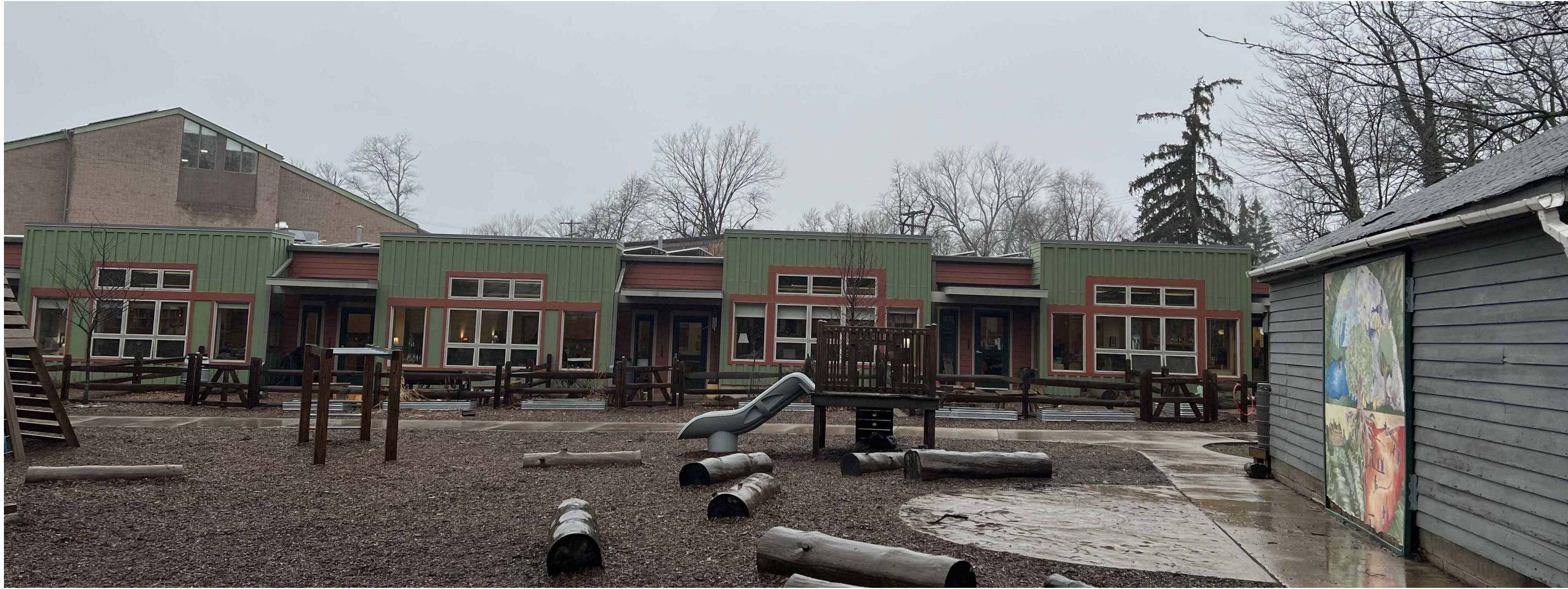
Q (NEIGHBORING RUFFING SCHOOL BUILDING)
