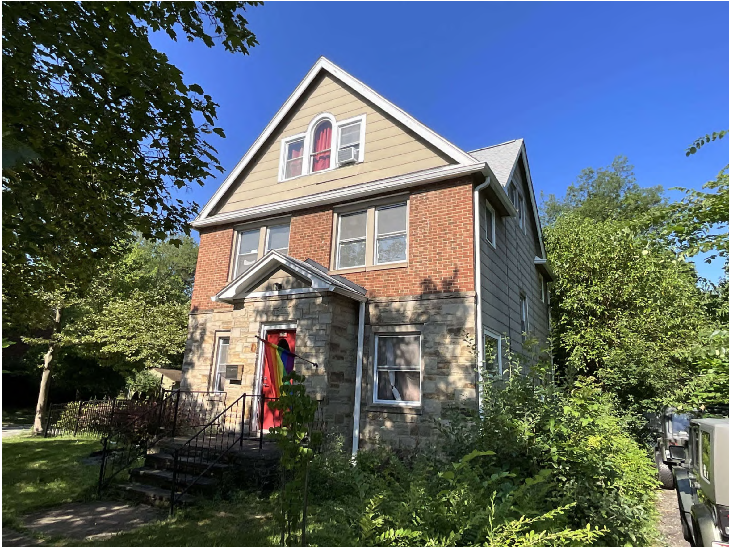
PHOTO 02 (2025-09-09) 2564 S. Taylor Road, OHIO 44118
