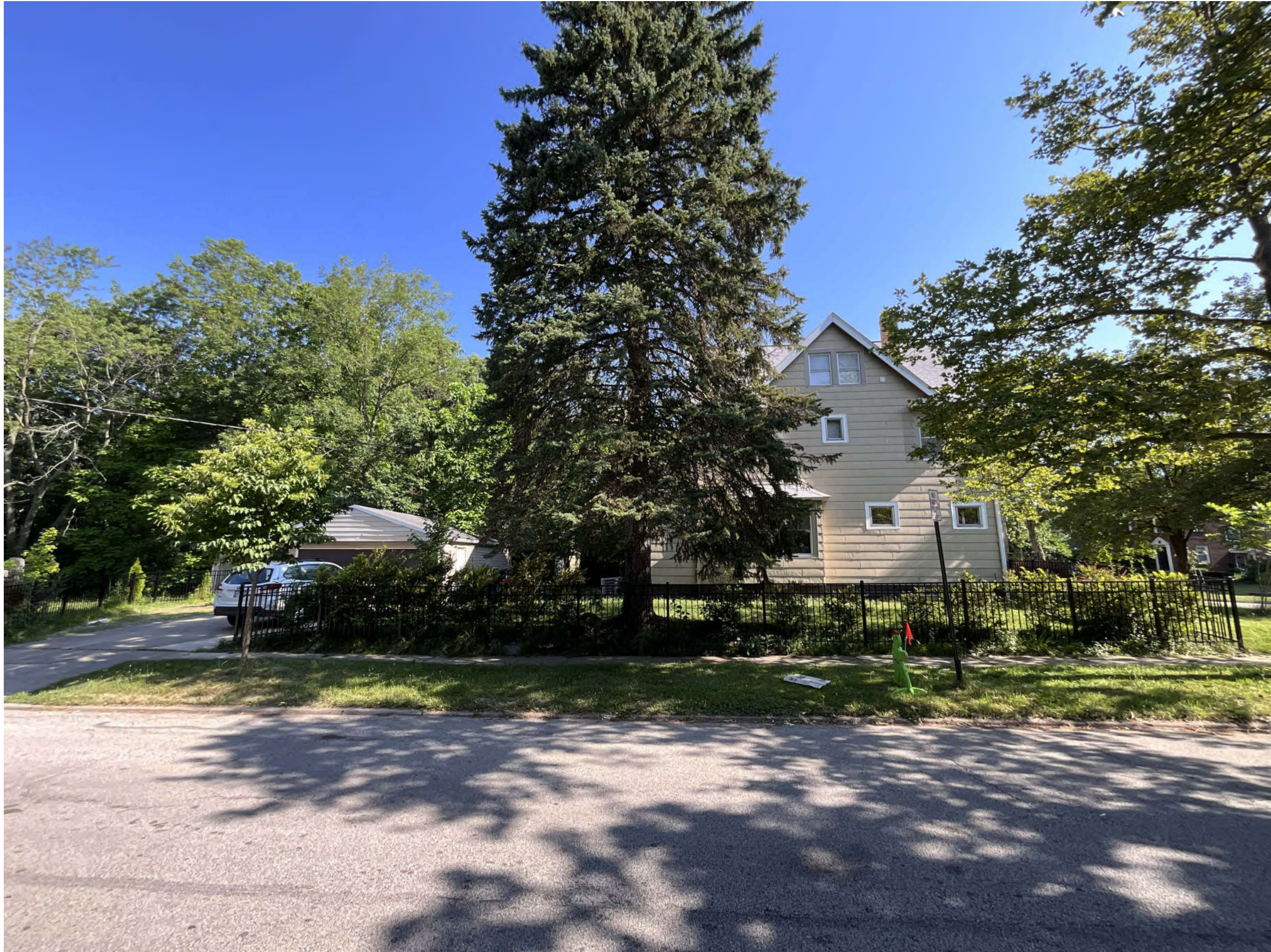
PHOTO 04 (2025-09-09) 2564 S. Taylor Road, OHIO 44118
