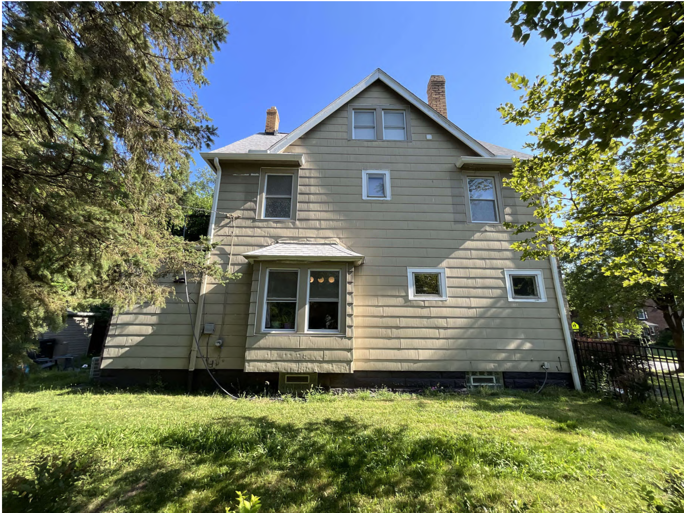
PHOTO 05 (2025-09-09) 2564 S. Taylor Road, OHIO 44118
