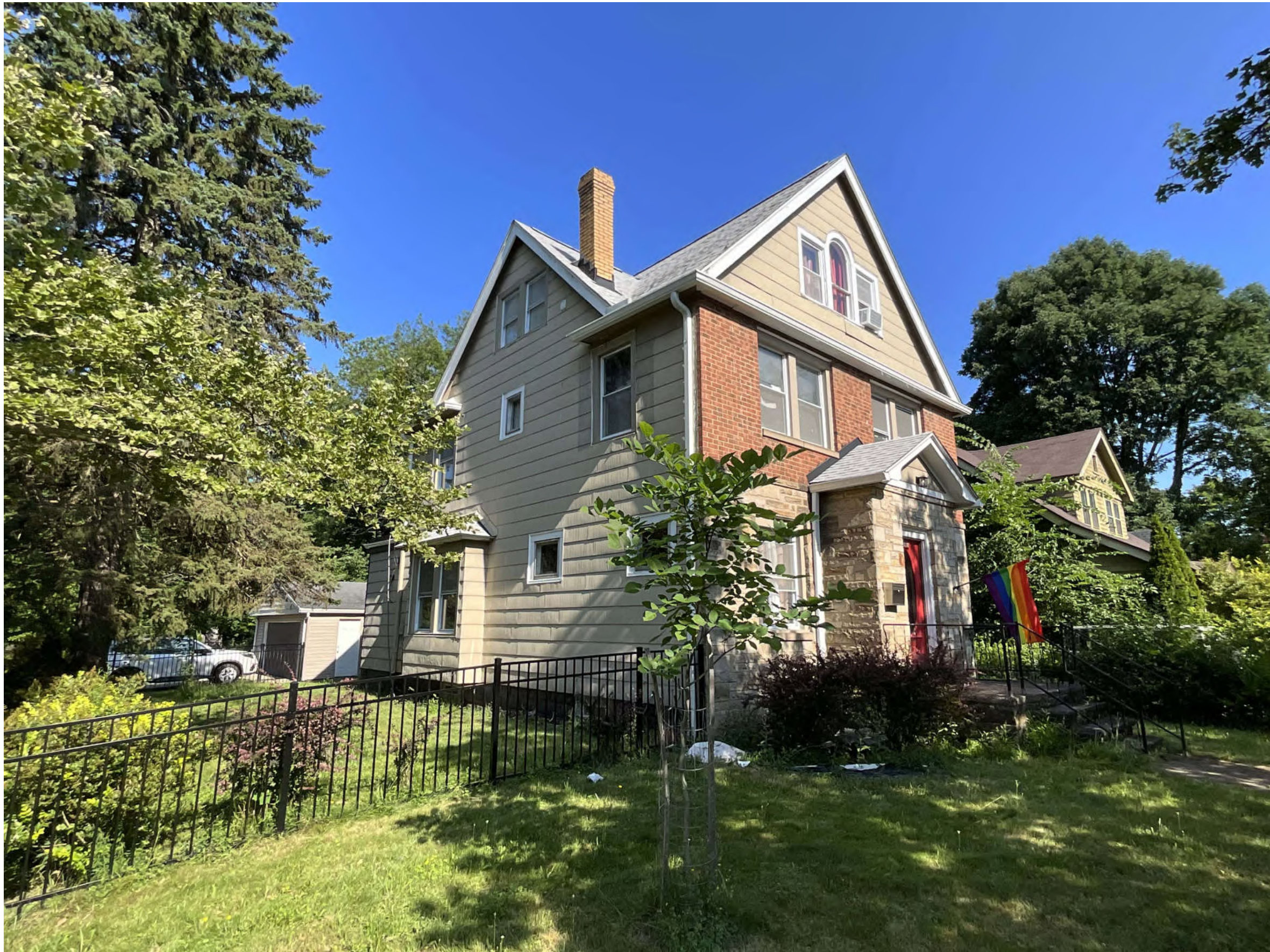
PHOTO 03 (2025-09-09) 2564 S. Taylor Road, OHIO 44118
