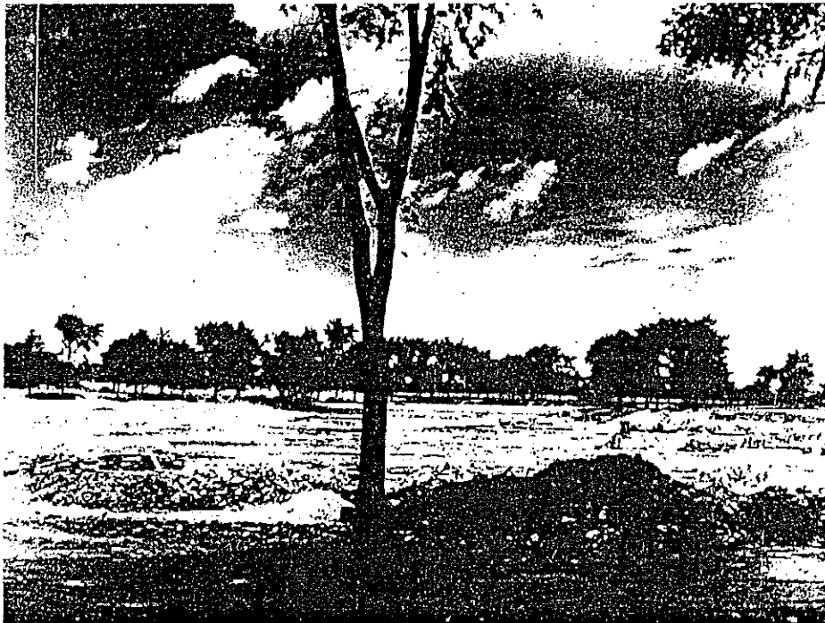
The lake under construction, which will cover five acres, doubling the size of the original lake at the Rockefeller Estate (CPL/1939).
