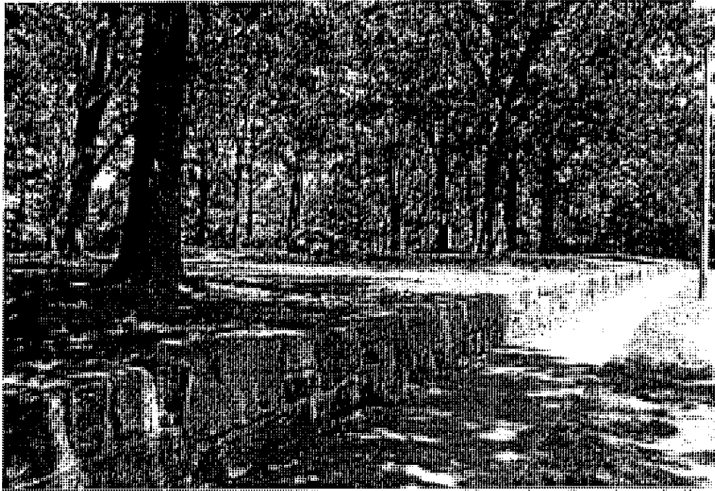
Low stone perimeter wall at Franklin Park in Boston, Massachusetts acts as both a retaining and free standing feature.
