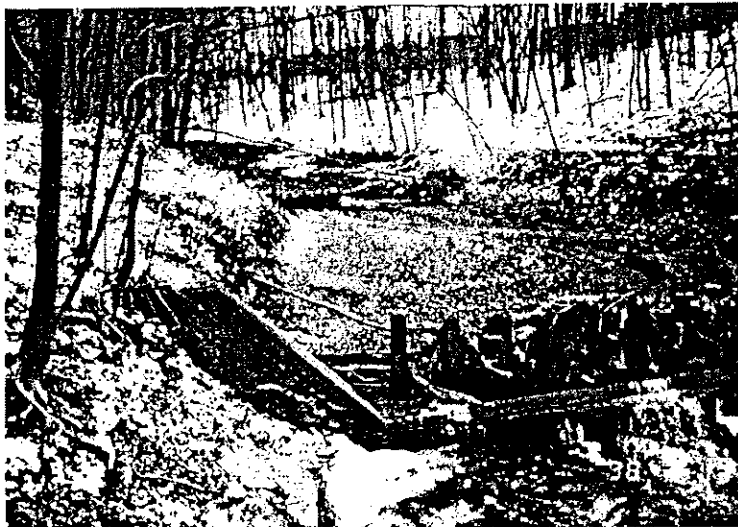
Rear and forward H-pile trash racks at Dugway Brook, 1998.
