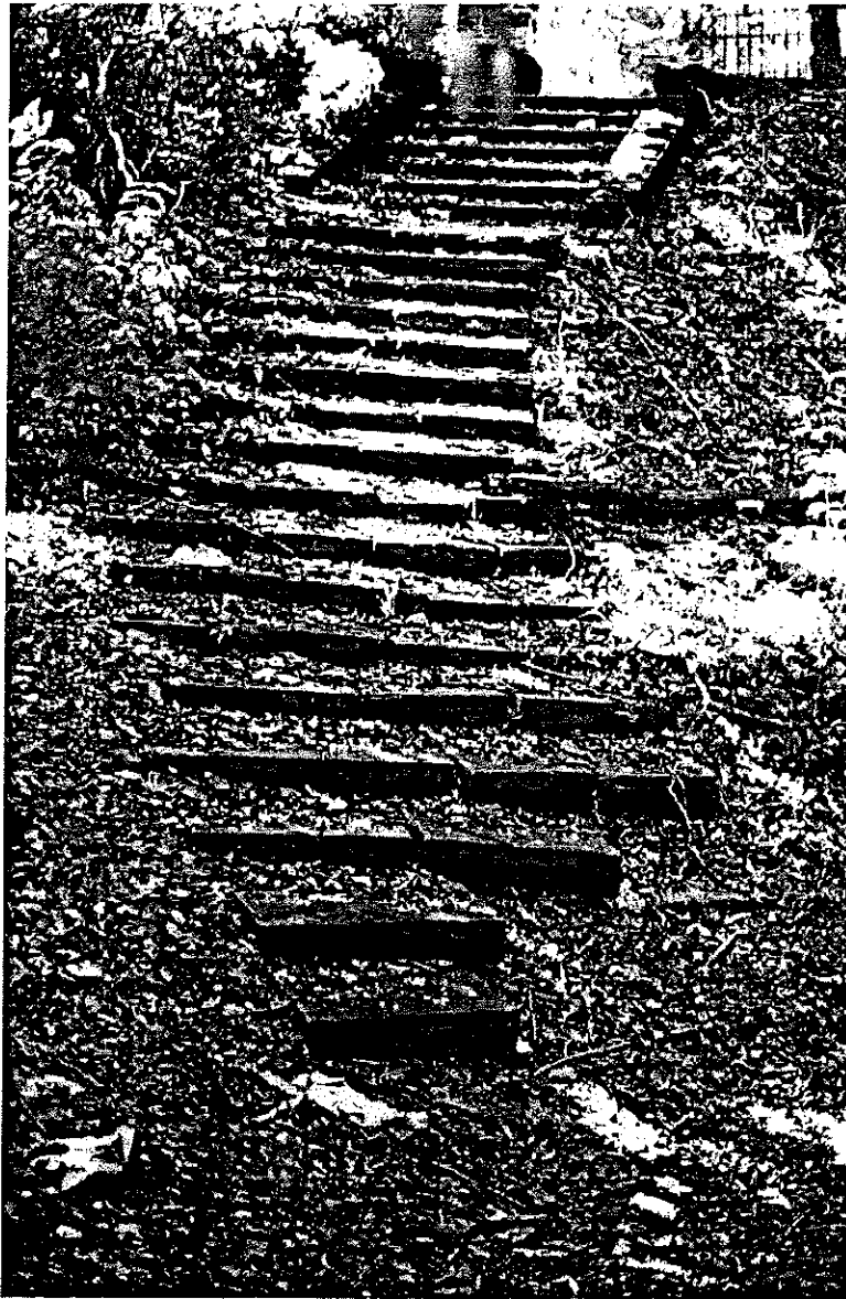
Stone steps at the trail from Superior Boulevard to the Dugway Valley picnic area, 1998.
