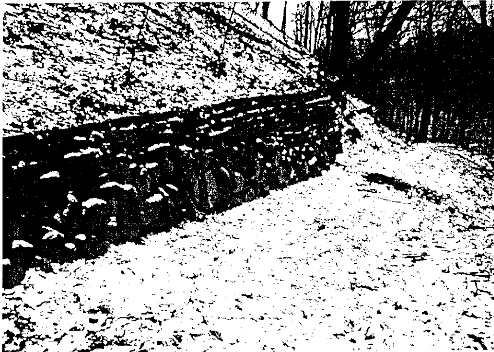
Stone terrace retaining wall at carriage drive, 1998.
