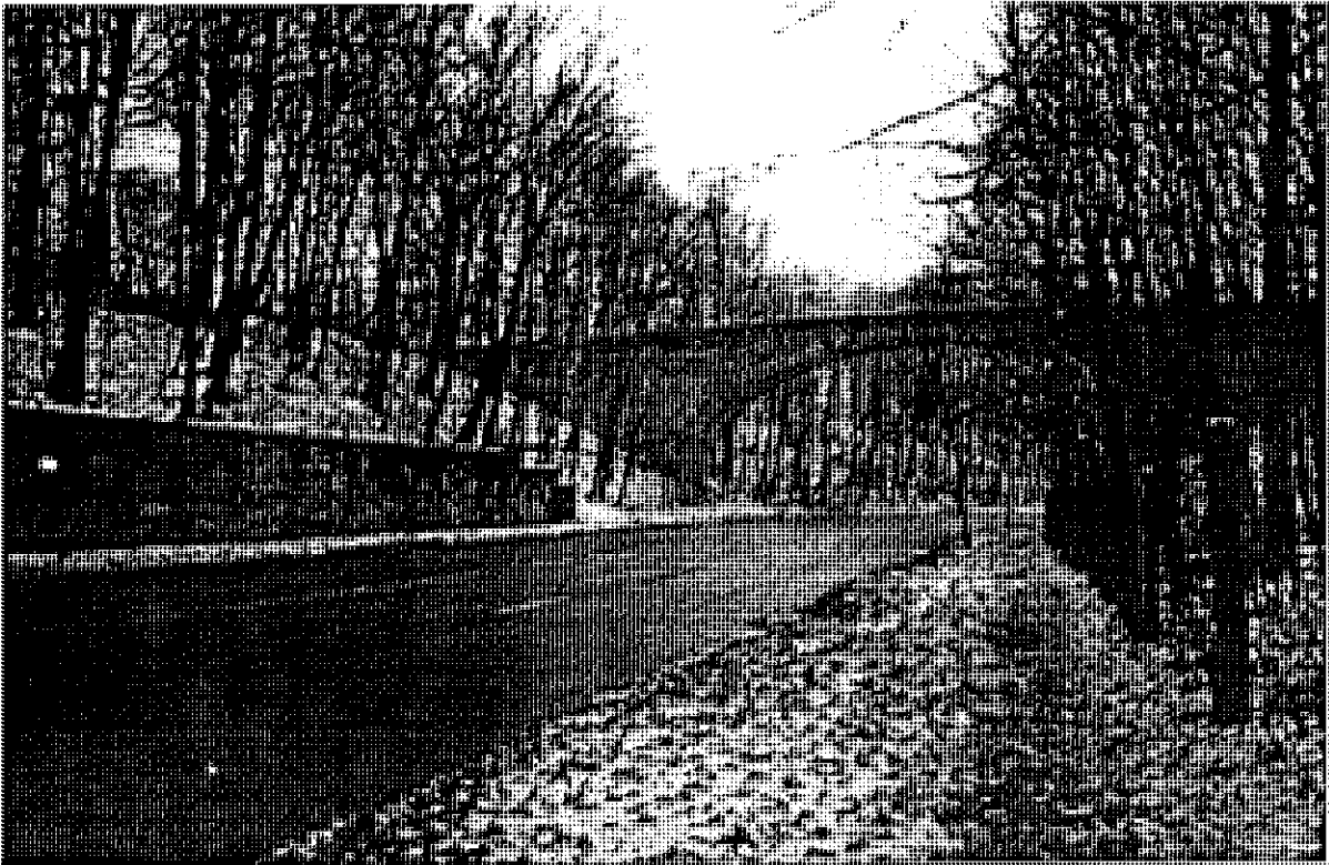
Forest Hill Boulevard Footbridge, 1968.
