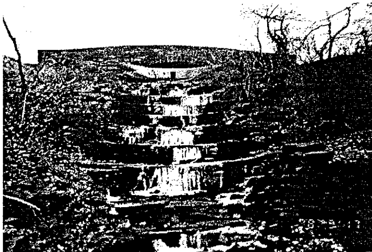
Stone stepped spillway at Lake, 1998.
