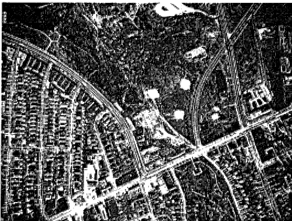
Work completed at Mayfield Road, Superior Road, Monticello Boulevard, and Lee Boulevard. (CHCH 1949).
