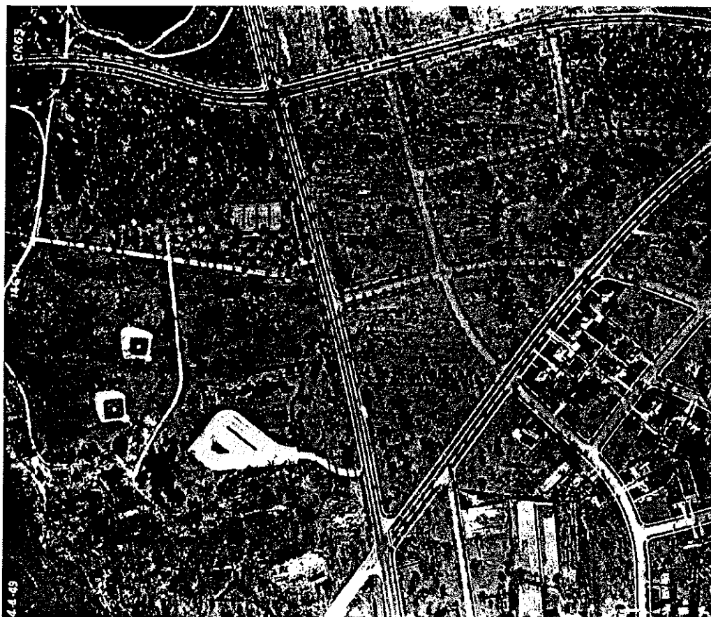
Work completed at Lee Boulevard and Monticello Boulevard. (CHCH 1949).
