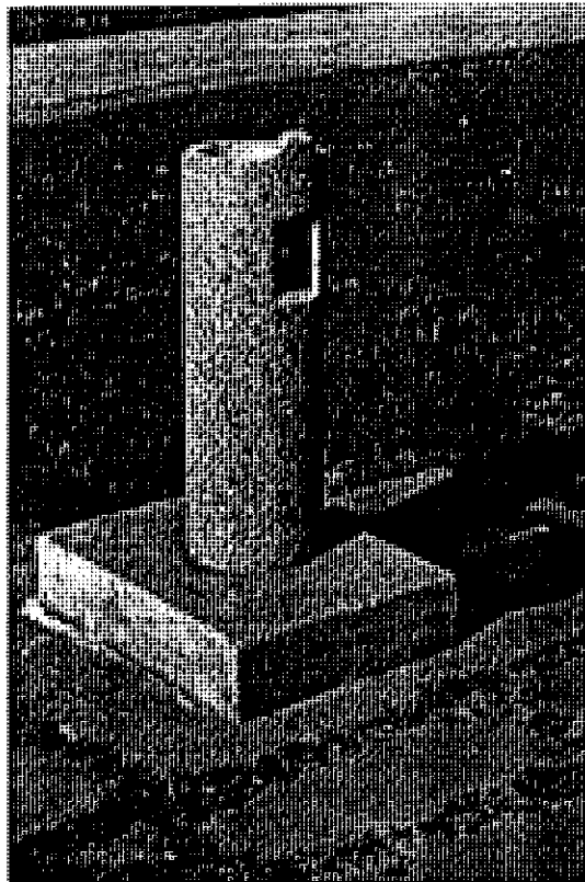
Inoperable water fountain, 1997.
