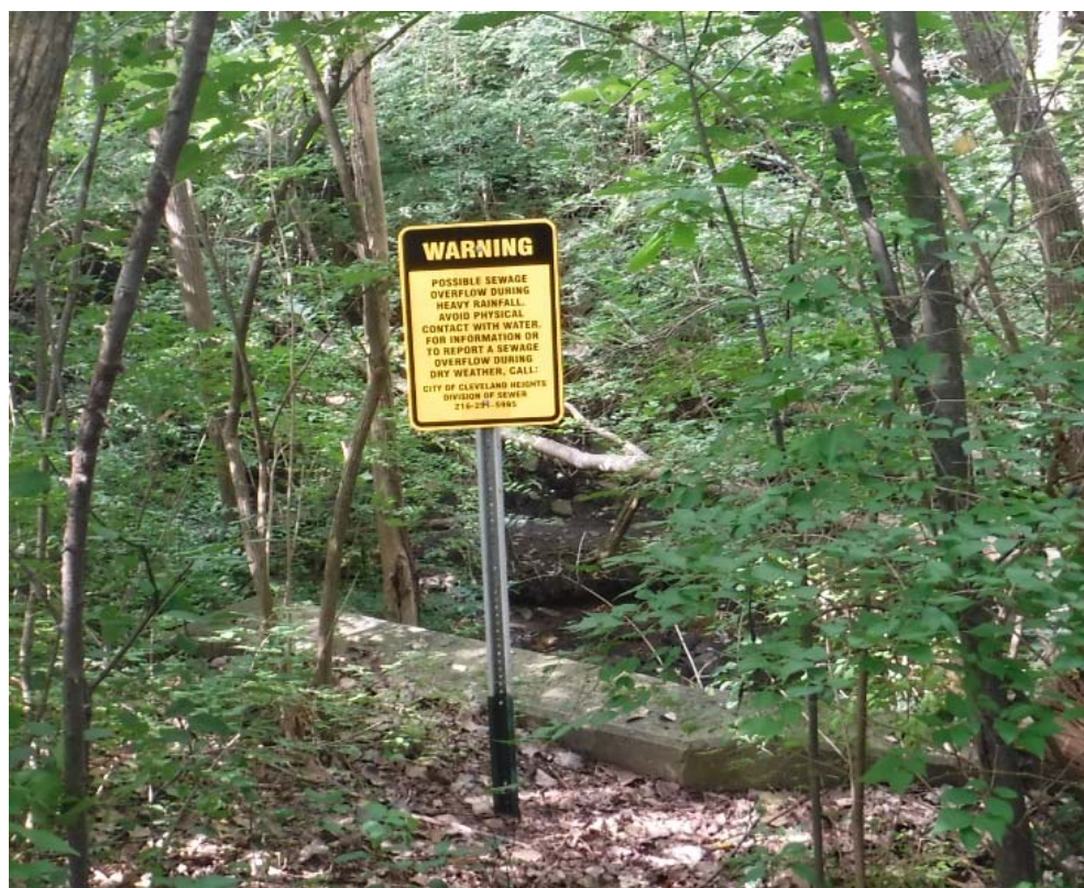
Figure 1. Example Signage Warning of Potential Wet Weather Overflow
