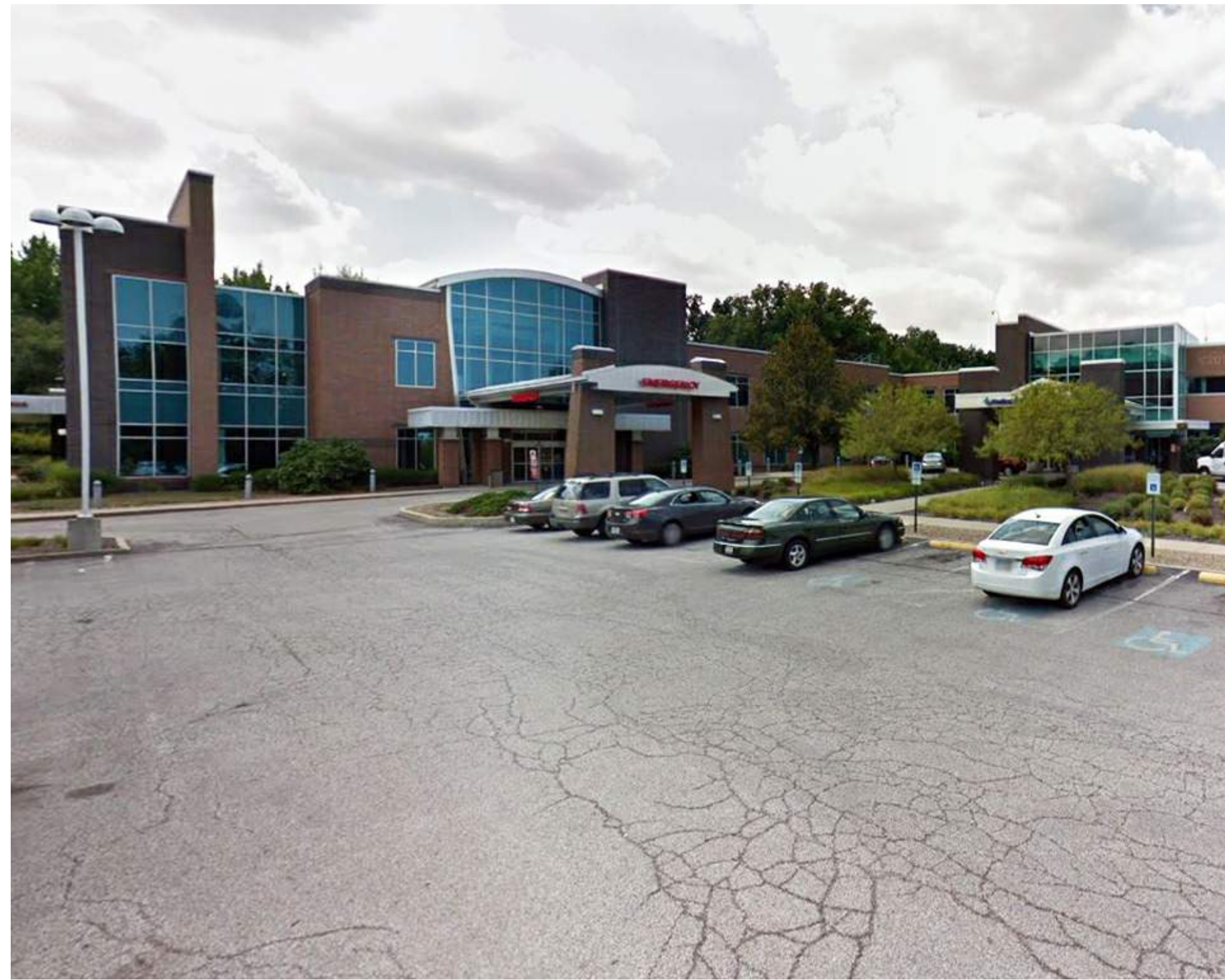
VIEW OF EMERGENCY DEPARTMENT AND OFFICE BUILDING FROM PARKING AREA
