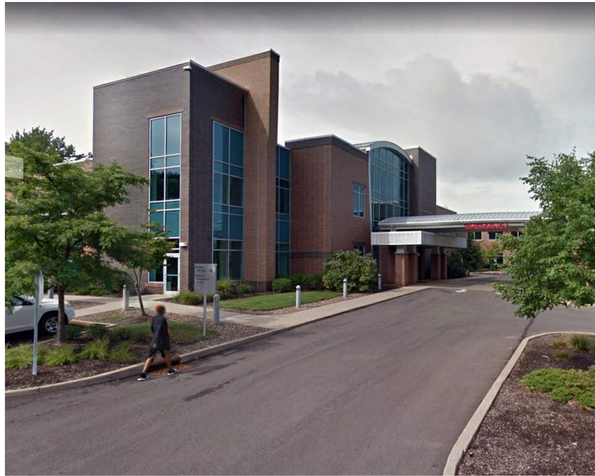
VIEW OF EMERGENCY DEPARTMENT ENTRANCE AREA
