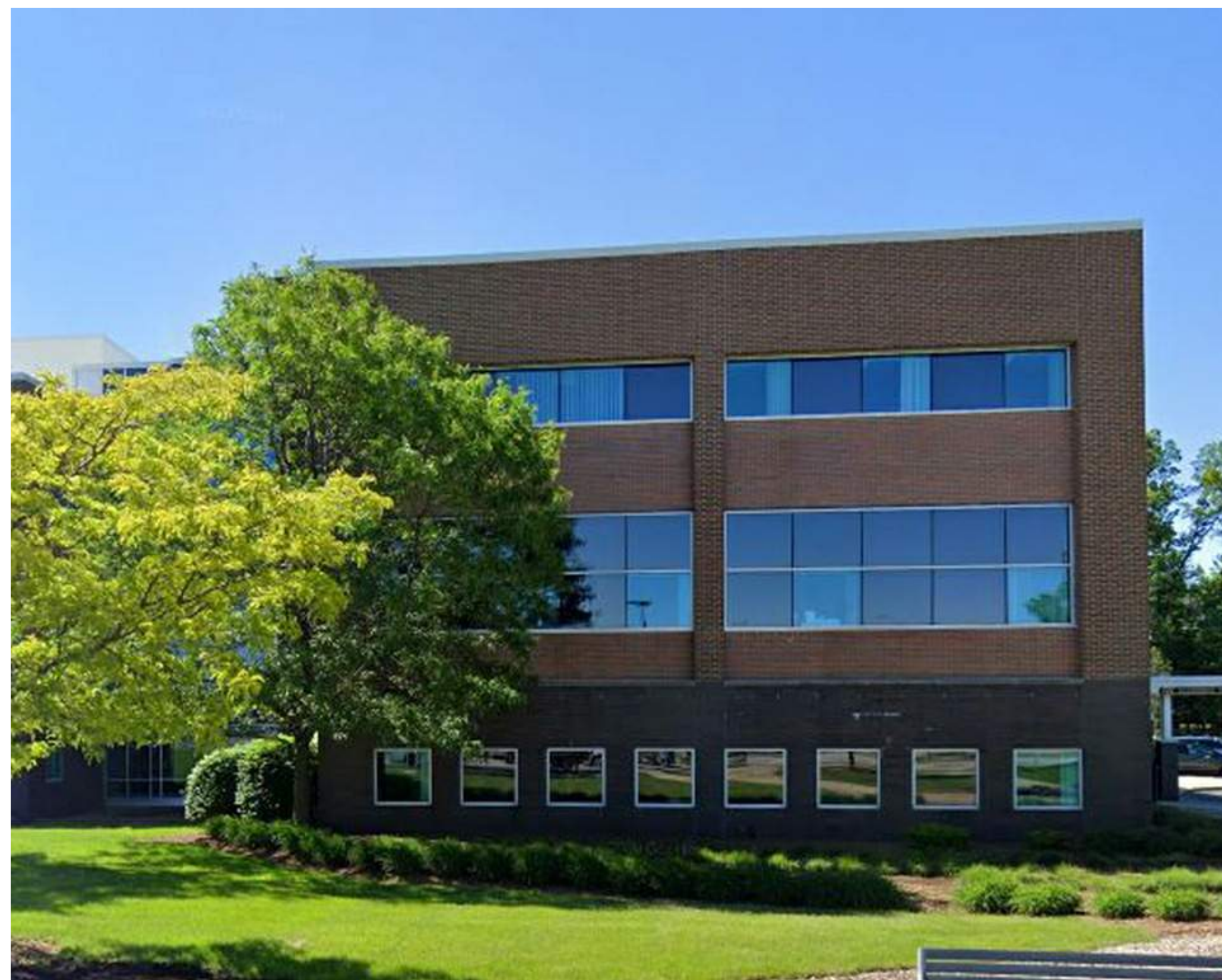
VIEW OF OFFICE BUILDING FROM SEVERANCE CIRCLE
