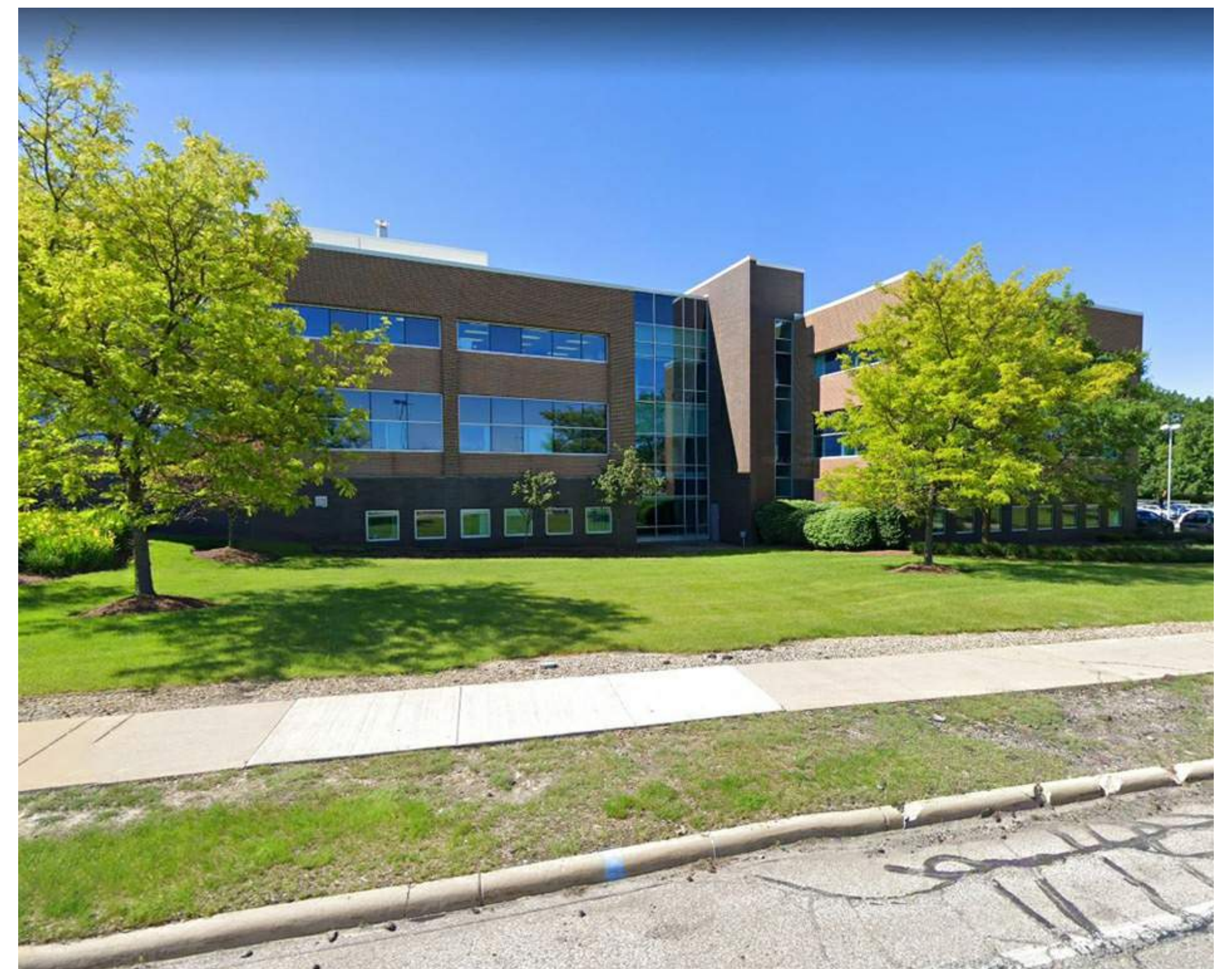
VIEW OF OFFICE BUILDING FROM SEVERANCE CIRCLE
