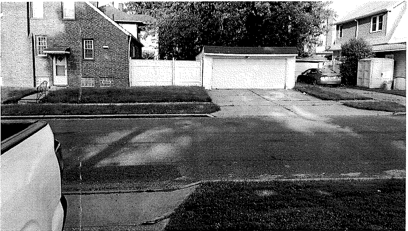
Minor Park - View East side of street
