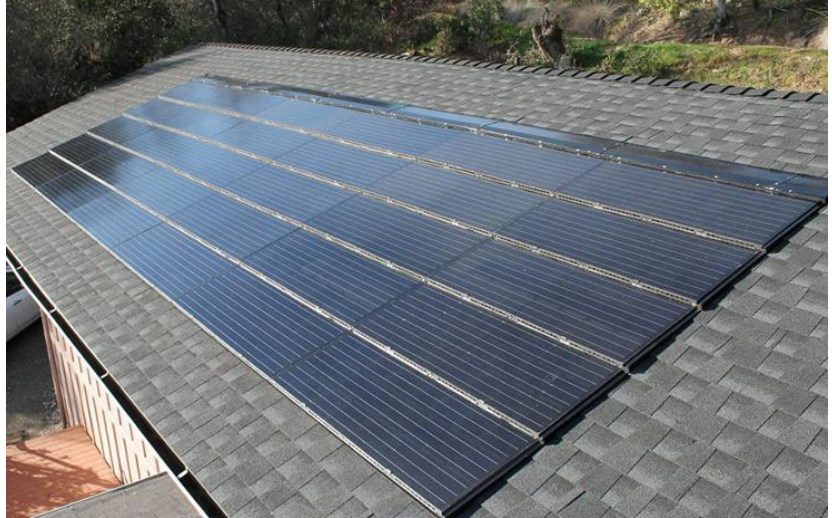
Roof Mounted Low Profile Solar Collector
