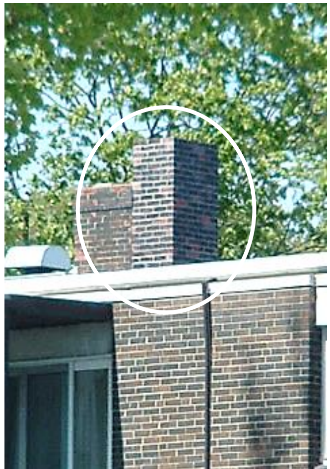
Fiberglass Chimney Shroud
